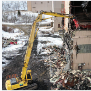
High Reach Demolition Equipment
